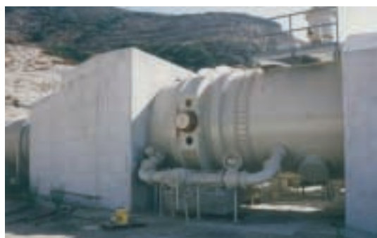
Emergency shut down valve 3650 mm / 144 inches for a hydroelectric power unit
