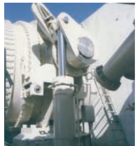
Hydraulic cylinder for a hydroelectric power unit
