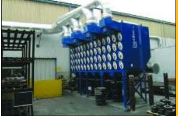
DFO 4-112 on titanium grinding
